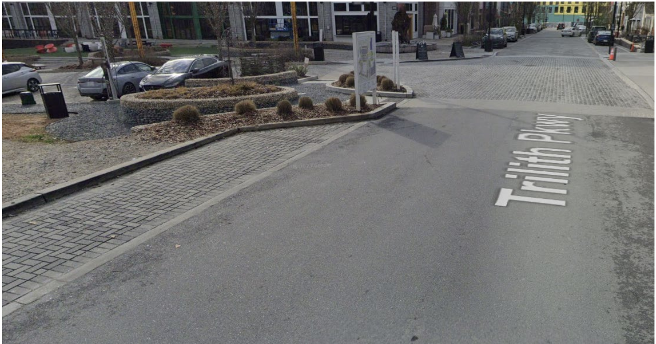
Example of Vehicular Pavers/Stamped Concrete at On-Street/Parallel Parking, Trilith Pkwy, Fayetteville, GA
