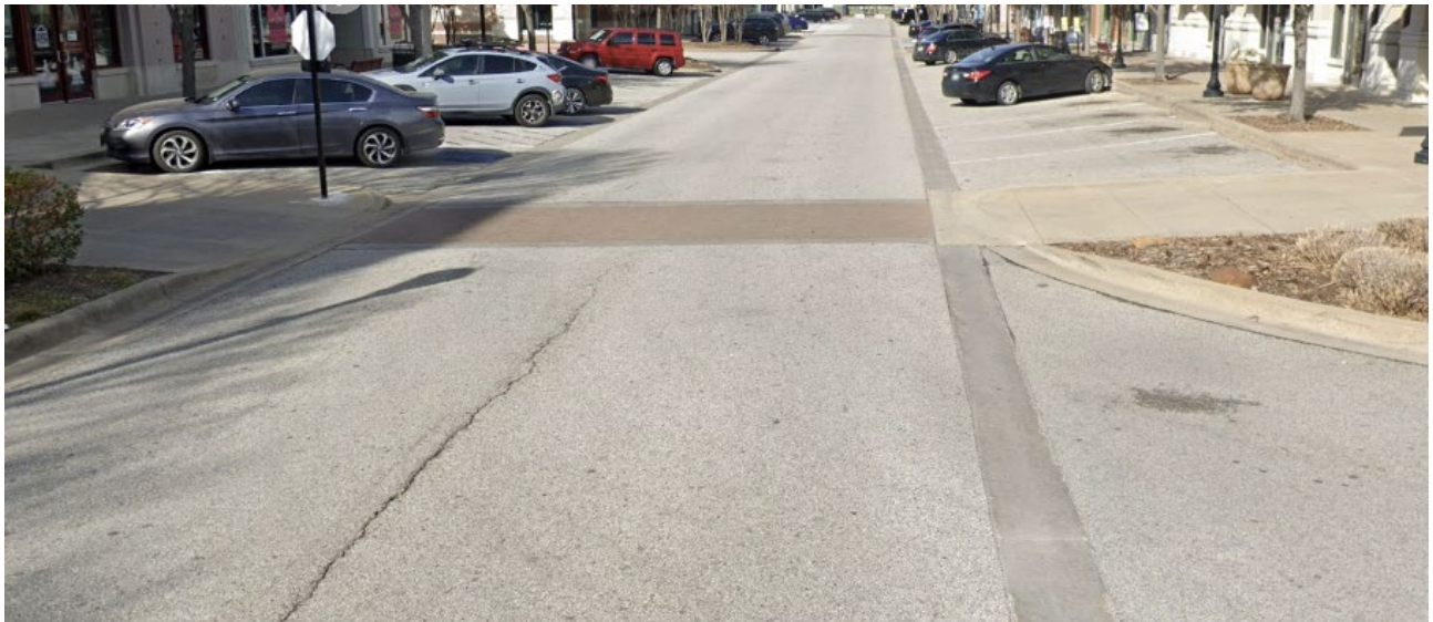
Example of Vehicular Pavers/Stamped Concrete at Pedestrian Crosswalk, Firewheel Town Center, Garland, TX
