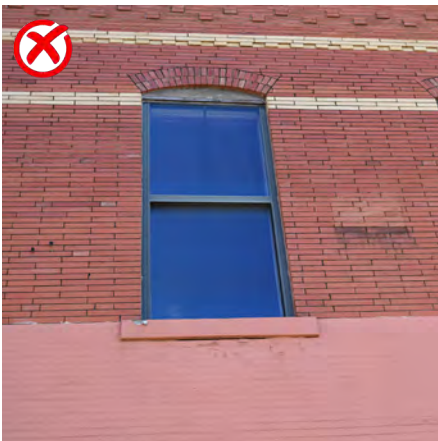
Replicate the character of historic sash divisions in a replacement window. The top image shows an original double-sash wood window from 1900, divided into two panes in each sash.
