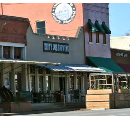
Although the parapet on this modern storefront resembles the parapet of an older building in the same location, the storefront elements (bulkheads, display windows, doors and transoms) are distinguishable as new construction.
