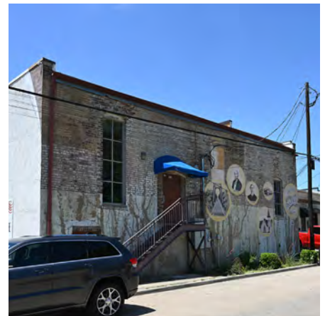
Incorporate window and door openings at a similar solid-to-void ratio, proportion and alignment as those on similar buildings. The windows and door on this addition are similar to the neighboring buildings.
