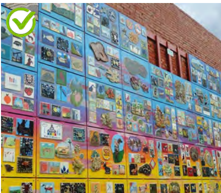
Paint or print murals on canvas or panels. These panels are affixed to an unpainted brick wall using a wood frame.
