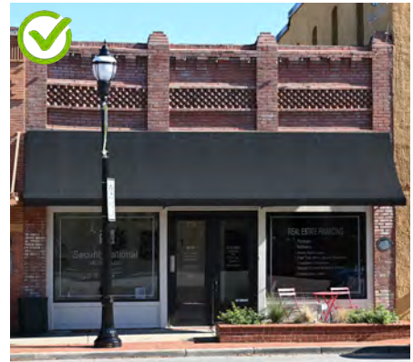
This storefront is a simple interpretation of the original. The arrangement of the windows and doors follows the established ratios and scale of other historic buildings on the block.
