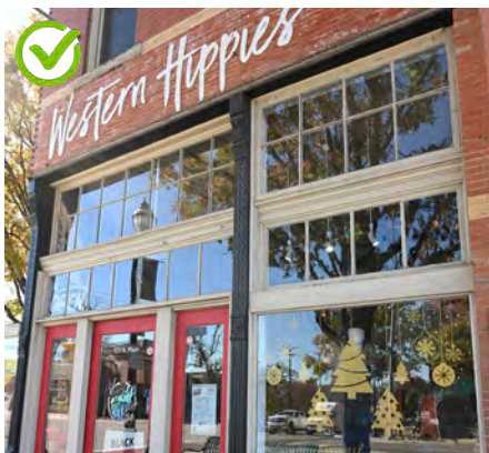
Preserve key historic features like these transom windows.
