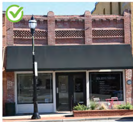
These wood bulkheads are simplified interpretations of the originals, seen in the top photograph. They keep the proportions and character of historic bulkheads.
