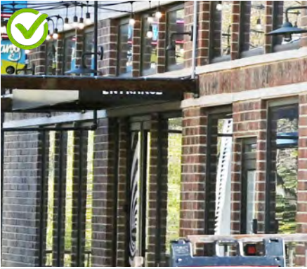
Incorporate a bulkhead, display window and transom in a new storefront design. New designs for windows, storefronts and architectural features provide visual interest while indicating that the building is new.
