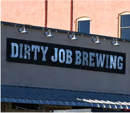
Direct lighting towards a sign from external, shielded lamps.
