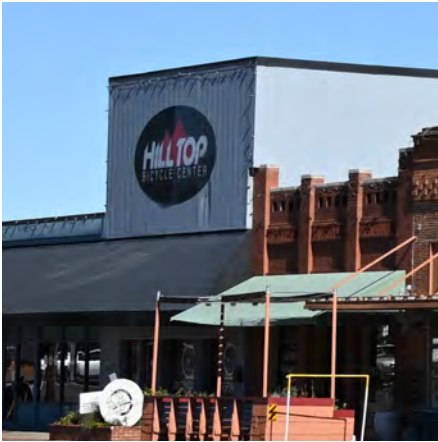
Consider removing non-historic coverings and alterations as an initial phase. A rehabilitation of the 1894 Post Office Building might begin with the removal of the metal panel slipcover with the restoration of the storefront in a later phase.
