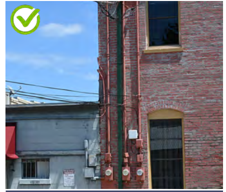
Locate utility lines and junction boxes on secondary and tertiary facades, and group them where possible. These electric meters are grouped together on the rear wall of this building.
