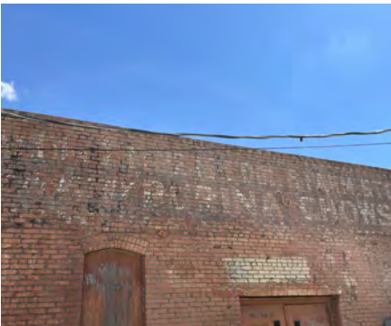
Historic painted wall signs, or "ghost signs" should be left exposed whenever possible, and should not be restored to the point that they no longer provide evidence of a building's age and historic function.
