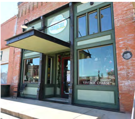
Design the awning or canopy to be in proportion to the building. This canopy fits within the doorway.
