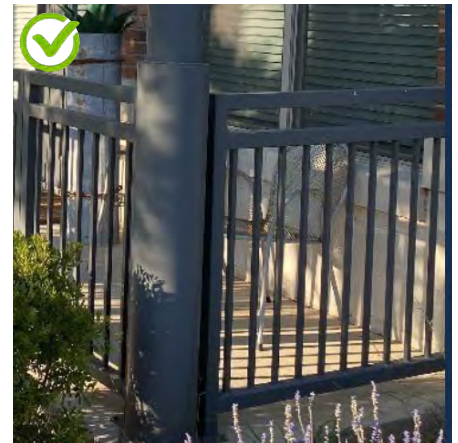
Simple metal and wood railings are appropriate. The railing should be mostly transparent.
