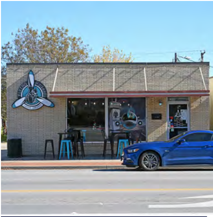
Restore a storefront to its original design based on its time period.
