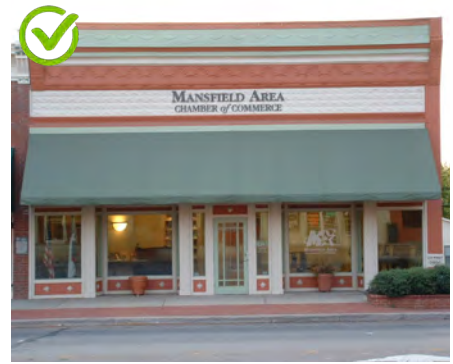
This reconstruction incorporates the elements of a traditional storefront, including display windows, bulkheads and transom windows.
