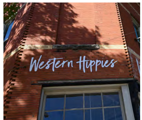
Example of a wall sign.
