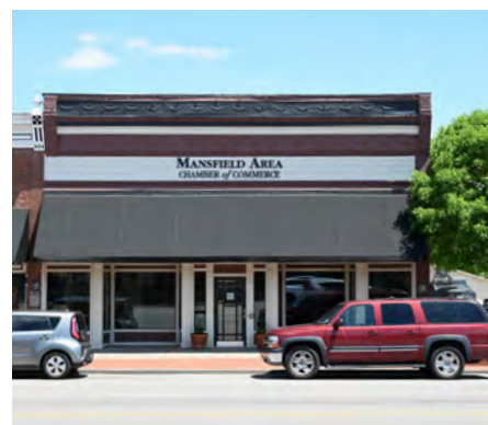
Mount a sign to fit within existing architectural features, such as the sign frame or sign band, using the shape of the sign to help reinforce the horizontal lines of the building.
