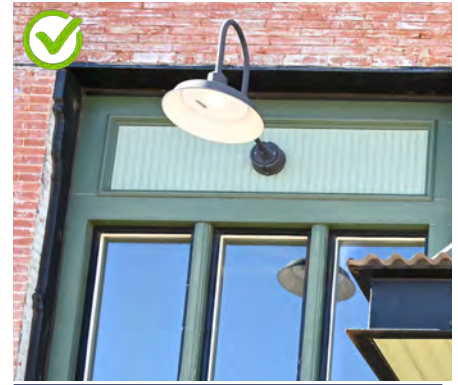
Use lighting fixtures that are appropriate to the building and its surroundings in terms of style, scale and intensity of illumination.
