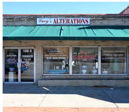
Flat canopies should be retained if present and replaced where needed. The flat canopy on this building was replaced with drop-front style awning.
