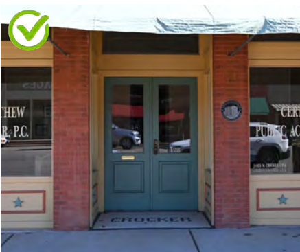
Consider recessing the primary entry door from the front façade to establish a distinct threshold for pedestrians, typically four feet.
