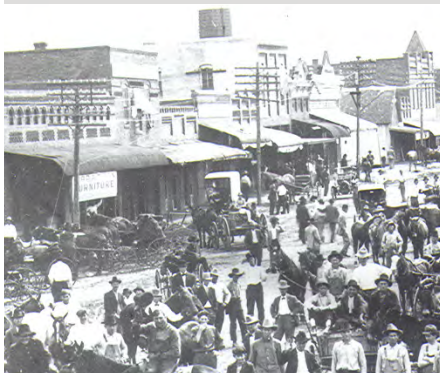
A variety of canopies can be seen in this 1907 photograph of Water Street. Examples of shed roof and flat canopies can be seen on the buildings. Note the awning on the upper floor window on the second building from left.
