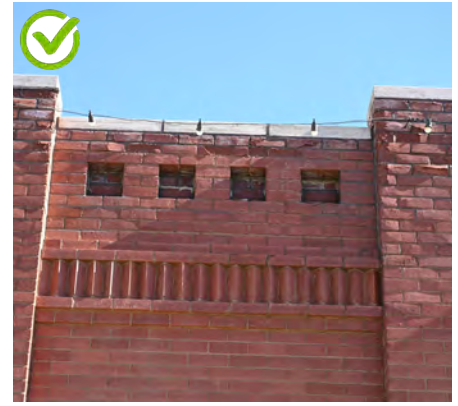
Preserve the parapet walls, cornices and decorative brick-patterning that characterize the building. During restoration of the storefront, the materials on this upper wall were retained.
