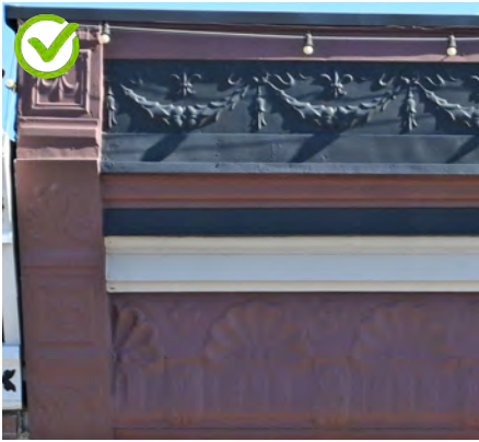
Preserve significant stylistic and character-defining features such as this stamped metal cornice.
