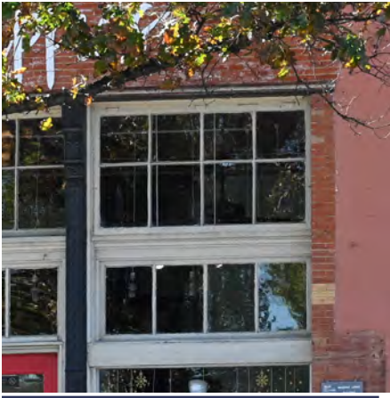
Do not remove, enclose or cover original transom window openings.
