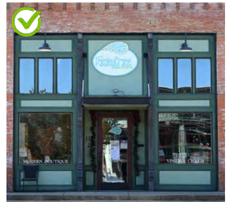
Where a historic feature cannot be repaired or restored, provide a design that is a compatible interpretation of the original. This reconstructed storefront keeps the form and scale of the original.
