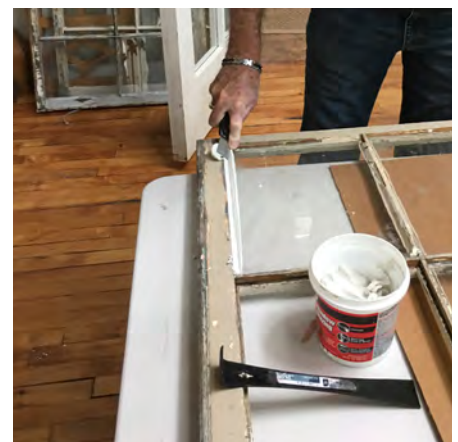
Preserve, retain and reuse early glass. Use putty appropriate to the window.
