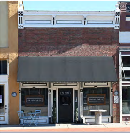
A minor trim color can be used to enhance the color scheme established by the major trim. The black paint on this building accentuates the appearance of the white base paint.
