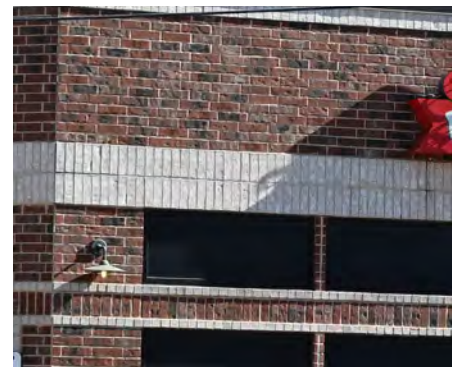
Use building materials appropriate to the surroundings. This red brick resembles the brick used on nearby historic buildings.
