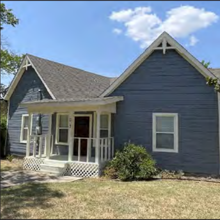
The Troy Hackler House c. 1880. This unusual house serves as an office for a financial advisor. The owner made substantial renovations in 2022, including replacement of the woodwork in the gables.
