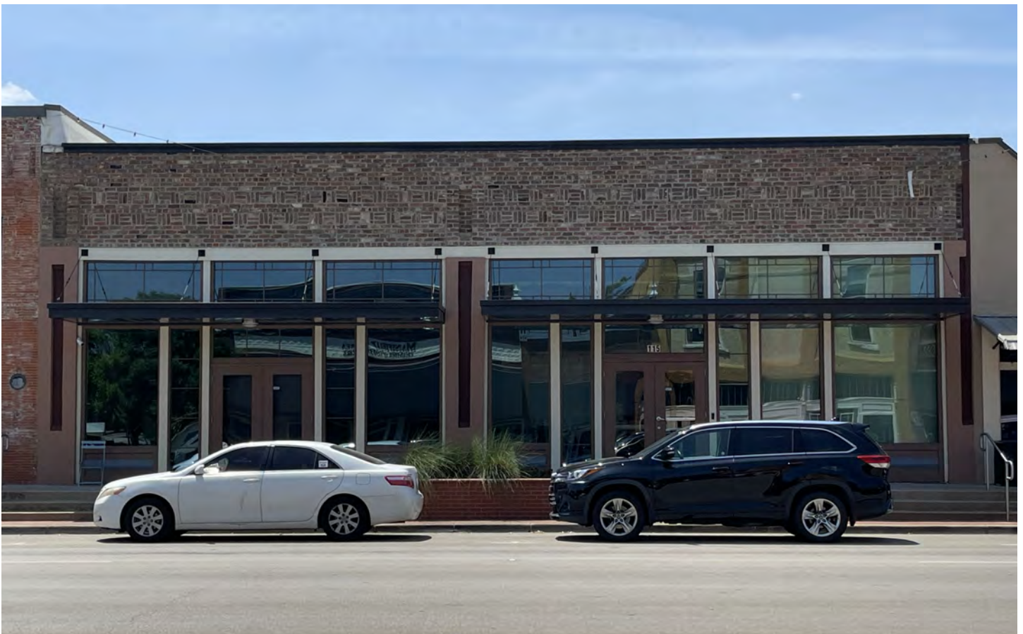
Top, the 1890 Dennis Mahoney Building in 2022 Bottom, the Mahoney Building after rehabilitation in 2023
