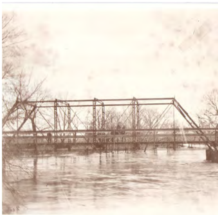
The North Street bridge washed away during the 1922 flood on Walnut Creek.
