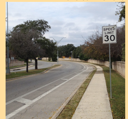
2-Lane Divided Roadway with Buffered Bike Lanes
