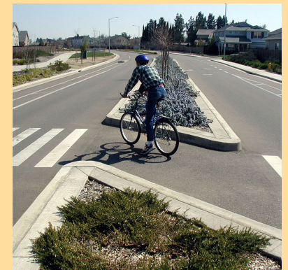
Median Refuge Island
