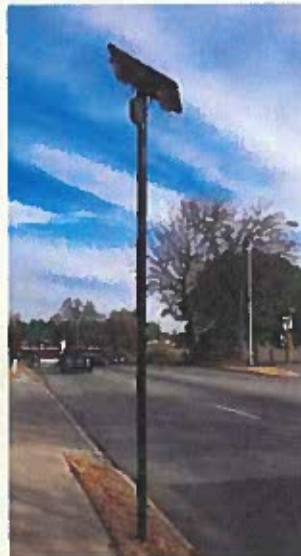
Solar & Flock Pole
