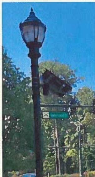
Solar & Existing Pole
