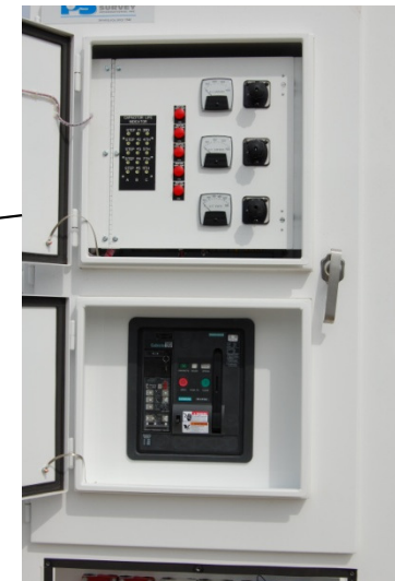
Main 600 V Electric Disconnect (behind panel) door
