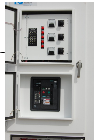
Main 600 V Electric Disconnect (behind panel) door
