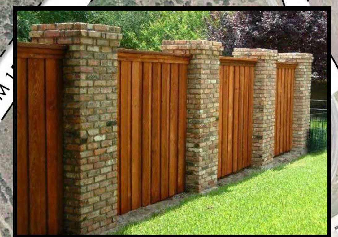
WOOD FENCE W/ MASONRY COLUMNS (COLUMNS SPACED PER PD)
