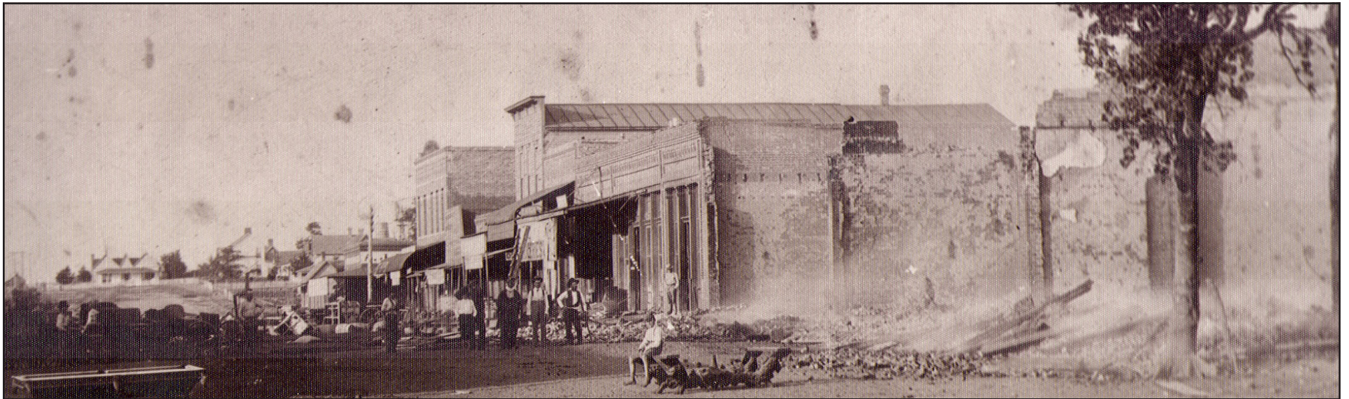
VIEW OF MAIN STREET AFTER THE 1901 FIRE. THE MAHONEY BUILDING IS THE FIRST UNDAMAGED BUILDING.
