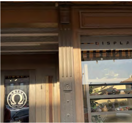
Where an architectural detail is missing or damaged beyond repair, alternate materials may be considered. This is a replica of a cast iron column that was removed from the building earlier.
