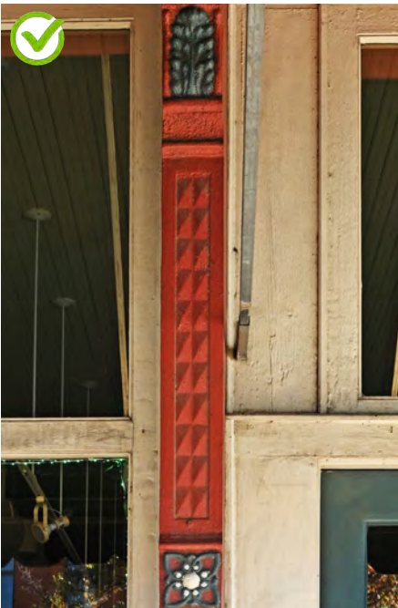
Maintain protective coatings like paint on exposed metals. The paint scheme on this column not only preserves a significant architectural feature of the building, but also highlights the column's decorative details.
