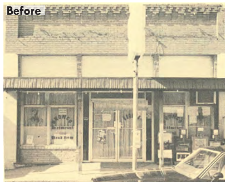
The original storefront of this building was removed during a modernization of the façade. The restoration involved a contemporary interpretation of the historic storefront.
