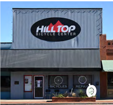
Consider removing any covering which obscures the original materials from view. This slipcover hides the upper story window openings and historic masonry.
