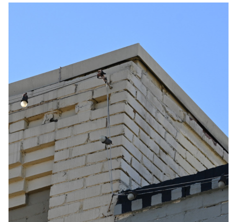
Inspect areas of the building that are exposed to weather or where water may gather, such as building parapets and roofs. This parapet shows signs of water damage.
