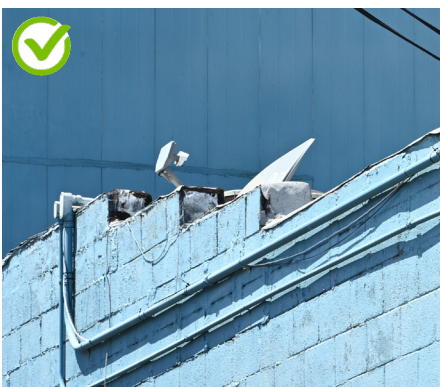
Locate satellite dishes and mechanical equipment out of public view. This dish is mounted on the rear of the building behind the parapet.
