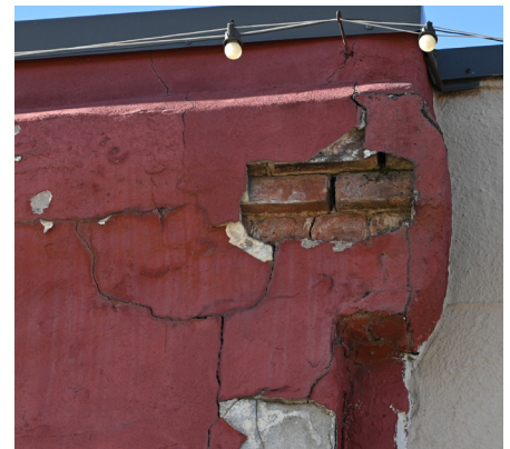
Remove coatings like paint and stucco from masonry surfaces if it can be done without damaging the masonry. It may be possible to remove the stucco from this parapet, but testing is necessary.
