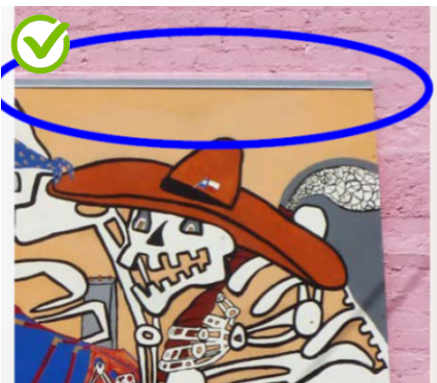
Prevent water from getting trapped behind the mural. The cap on this mural directs water away from the wall.
