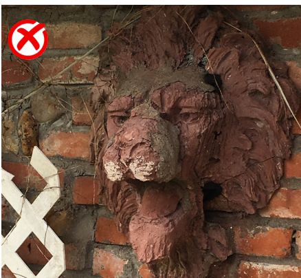
Do not remove architectural features that are in good shape or can be repaired. This lion's head ornamented a historic bank but was broken into pieces when it was removed from the building. The pieces were patched together with Portland cement, causing permanent damage to this feature.
