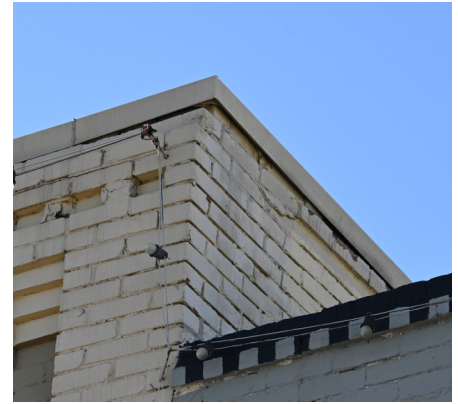
Applying paint or stucco to masonry can seal in moisture and cause damage to the material. The brick in this wall was damaged after water was trapped between the paint and brick.
