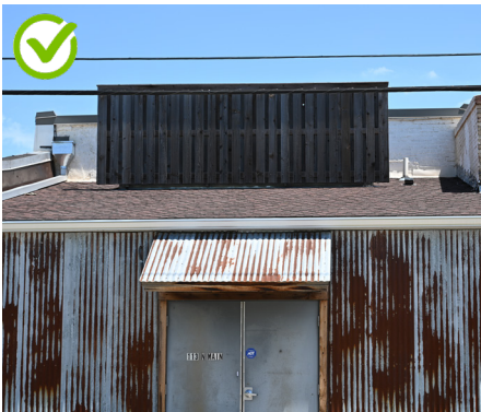
Screen equipment from public view. The roof-top HVAC units on this building are set back from the rear wall and screened by a board-on-board enclosure.
