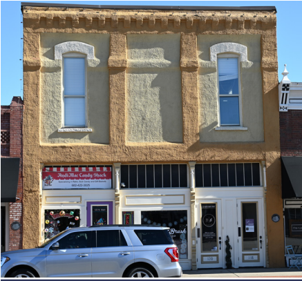
Stucco covers the masonry walls of this 1892 building. Removing the stucco must be done with care to avoid damaging the historic brick.
