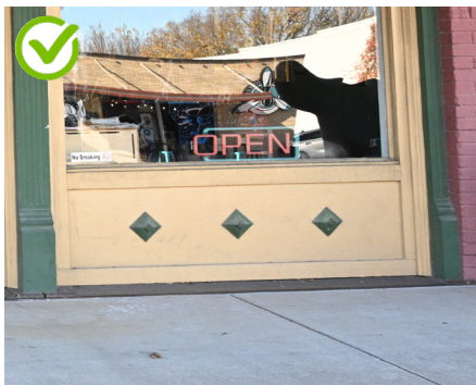
The wood bulkhead and the cast iron threshold seen here are important features of this historic storefront.
