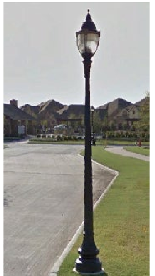
11' TALL ONCOR LIGHT STANDARD - AMERICAN POLE WITH FRISCO LUMINAIRE* (NOTE* THE ACORN LUMINAIRE MAYBE USED AS AN ALTERNATIVE TO THE FRISCO LUMINAIRE.)
