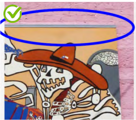
Prevent water from getting trapped behind the mural. The cap on this mural directs water away from the wall.
