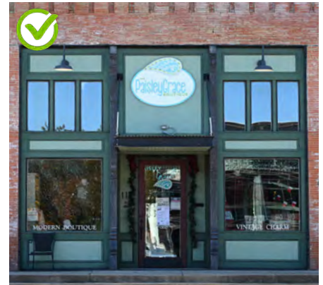
Where a historic feature cannot be repaired or restored, provide a design that is a compatible interpretation of the original. This reconstructed storefront keeps the form and scale of the original.
