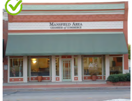
This reconstruction incorporates the elements of a traditional storefront, including display windows, bulkheads and transom windows.
