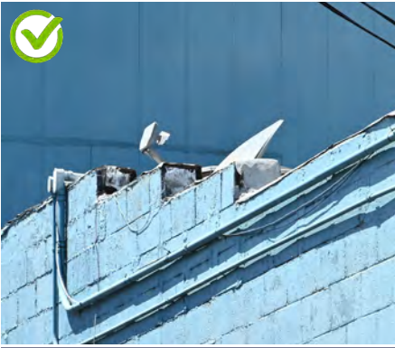
Locate satellite dishes and mechanical equipment out of public view. This dish is mounted on the rear of the building behind the parapet.
