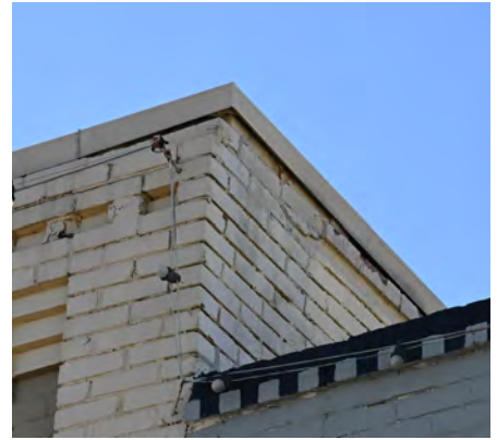
Applying paint or stucco to masonry can seal in moisture and cause damage to the material. The brick in this wall was damaged after water was trapped between the paint and brick.
