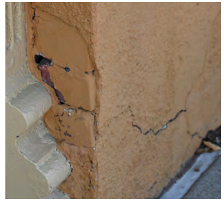
When this stucco deteriorated, the exposed brick was damaged by water. A maintenance plan can ensure that regular inspections and appropriate maintenance are carried out in a timely manner before major repairs are needed later.
