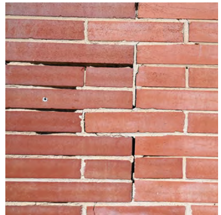
Repoint mortar joints where deterioration is evident, as seen on this section of wall.
