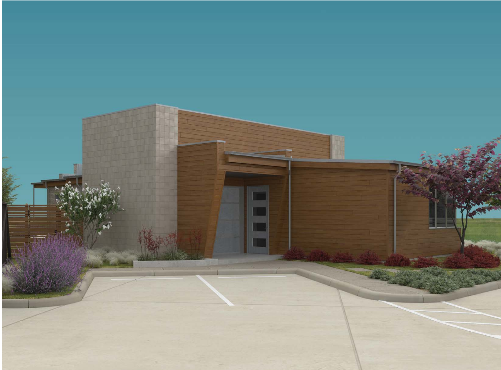
Building B - Entry
